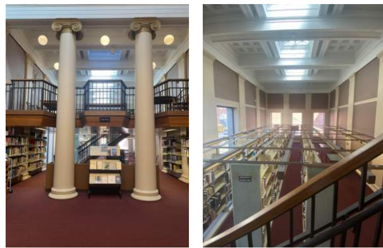
WEST WING SECOND LEVEL EXISTING CONDITIONS PHOTOS
