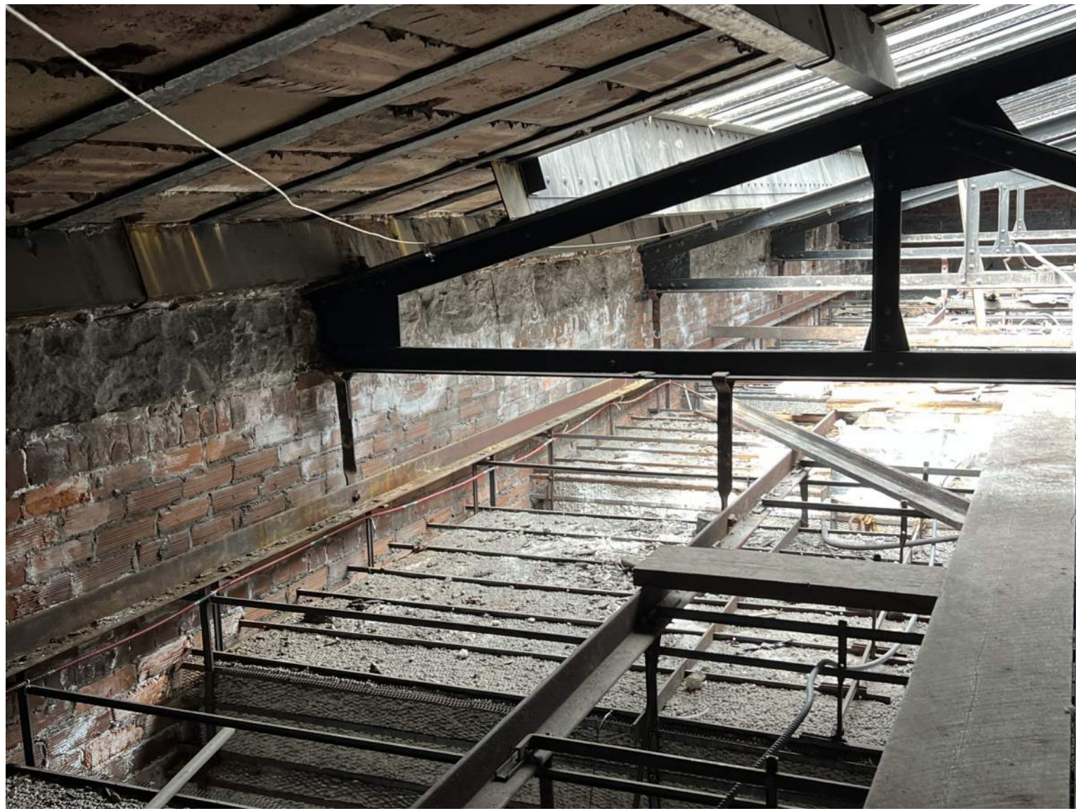
ATTIC TRUSS PHOTO, TYPICAL
