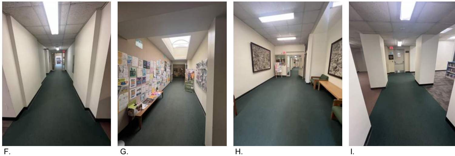
FIRST LEVEL CORRIDORS EXISTING CONDITIONS PHOTOS
