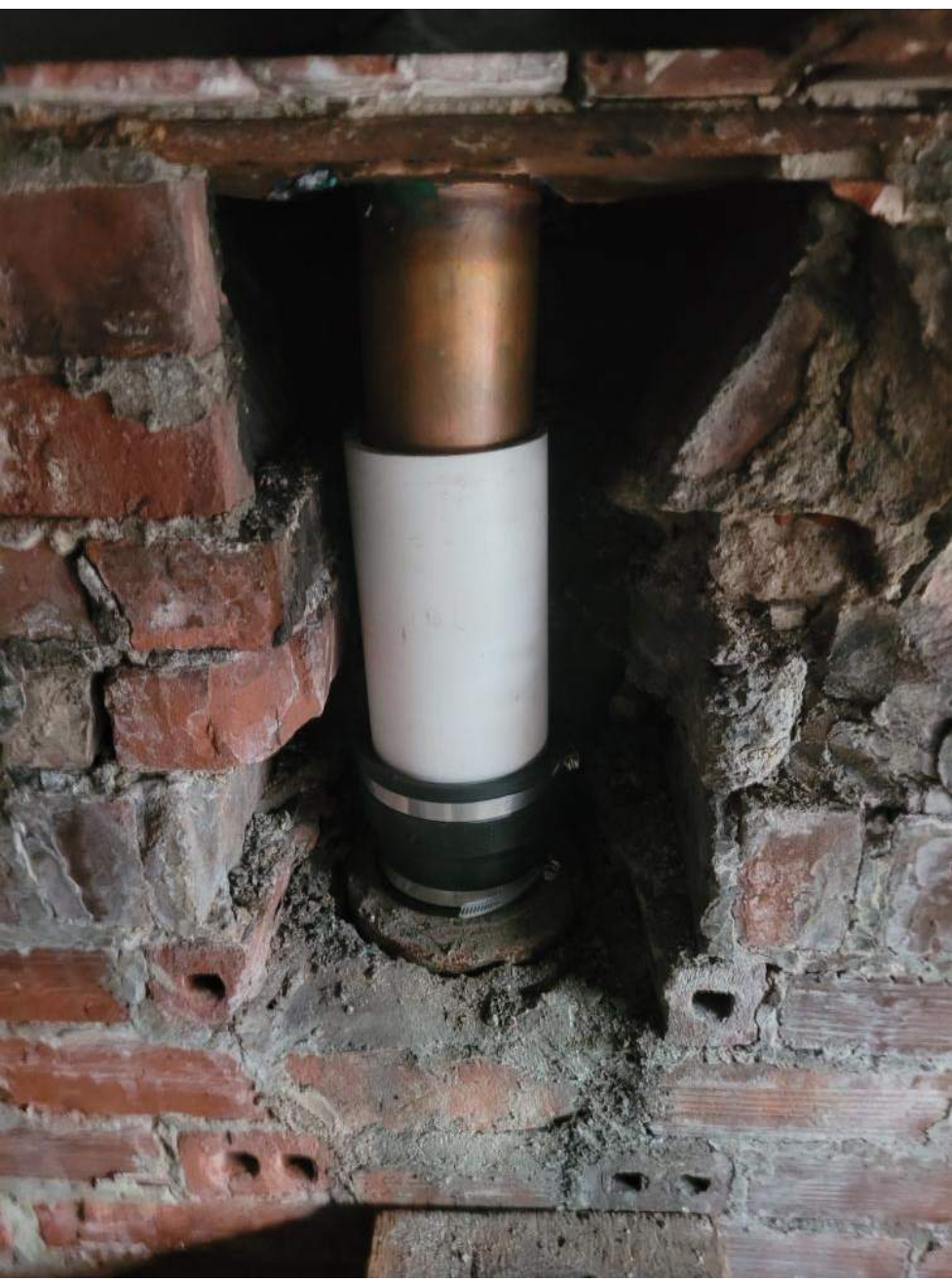
ATTIC DRAIN PHOTO, TYPICAL
