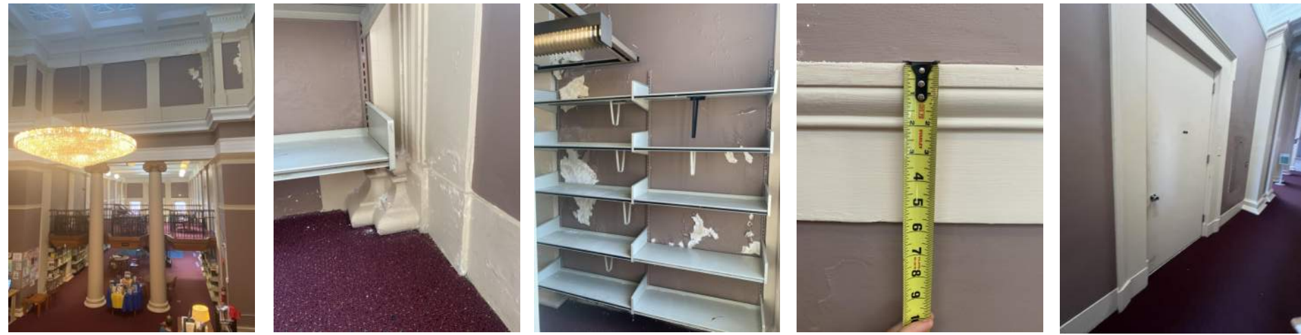
EXISTING CONDITIONS OF DETAIL ITEMS
