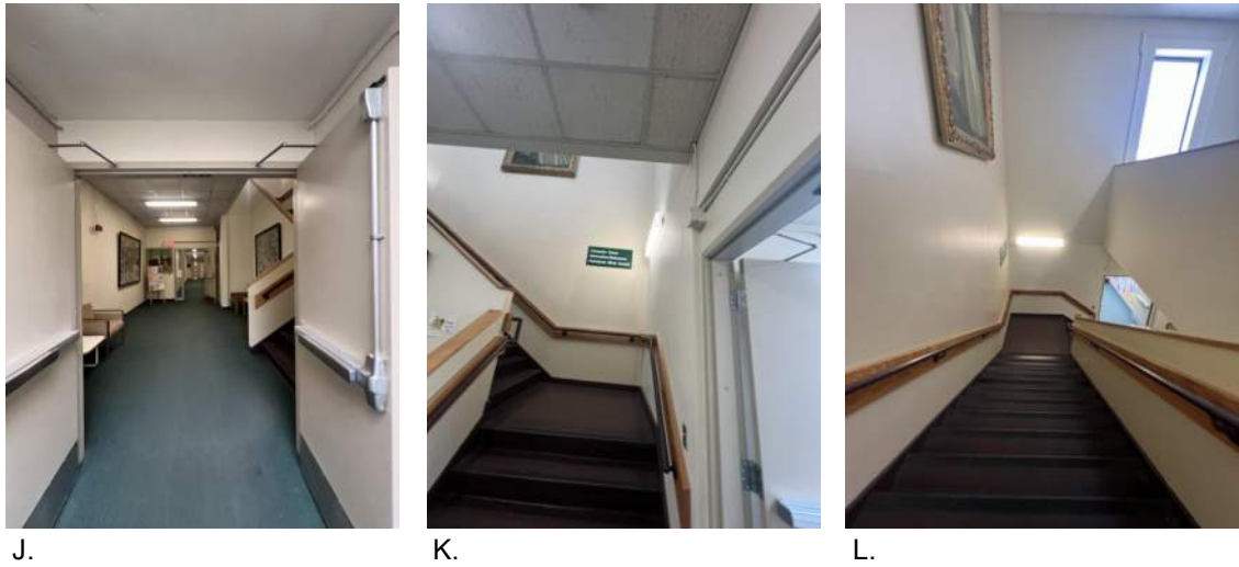
FIRST LEVEL MAIN STAIRCASE EXISTING CONDITIONS PHOTOS
