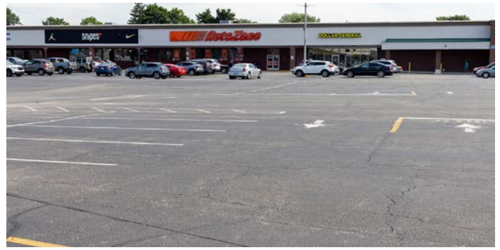
Excess impervious areas cause hotter temperatures and increased runoff. This parking lot could be retrofitted to add more trees, bioswales, and pervious surfaces that allow water to seep into the ground.
