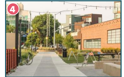
4 Provide off-street pedestrian/bike-only connection through former Apex property recently acquired by the City for redevelopment.
