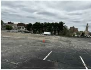
PHOTO 1: EXISTING 101 MAIN STREET PARCEL, REMAINS OF BUILDING FOUNDATION, RETAINING WALL, AND PARKING LOT.
