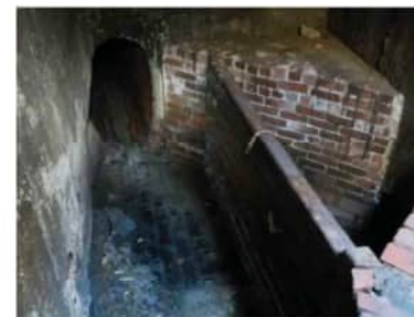
212 DIVERSION STRUCTURE (EX MH P210007) PHOTO 1: UPSTREAM COMBINED SEWER
